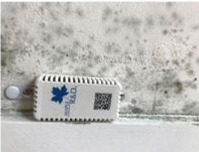
Such moisture related issues are dependant of water vapour production, ventilation, temperature and the thermal performance of walls and floors.
